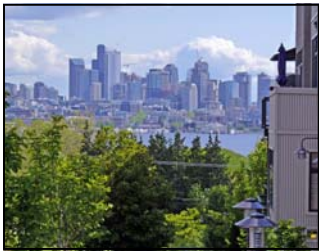
The view north over Lake Union of downtown Seattle shows a skyline with construction cranes in place although major new construction is winding down in 2010.
